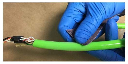
b Using the abrasive cloth, scuff the ends of the cable outer jackets.
