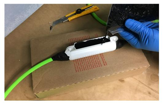
j Allow the compound to cure (from 16 to 36 hours, depending on the room temperature).
