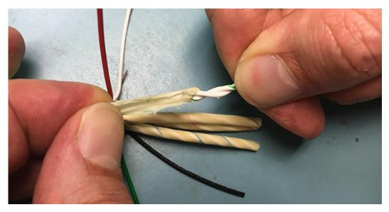
d Using the side cutters, cut each Ethernet pair to a different length so that there will be a 1/4" spacing between each wire splice.
