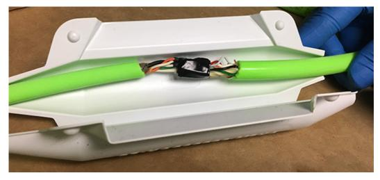
e Place the cable into the mold with the splice at the centre.
