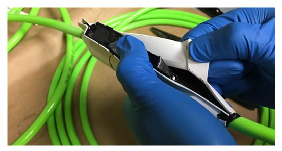
c Trim off the excess compound from the filler spout by cutting it off at the base.
